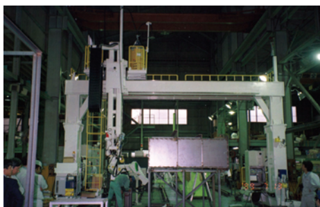
Fig. 9. General view of the welding robot equipment.
